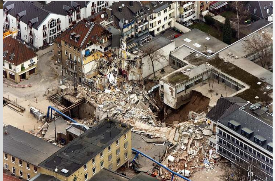
Monitoring omitted from this section of the works
